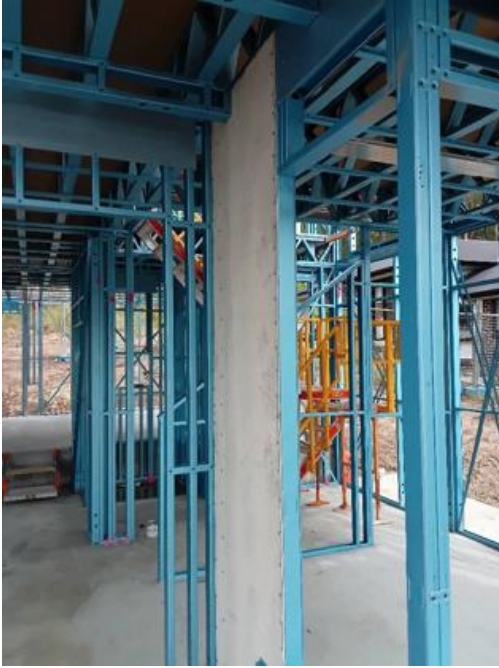
Typical sheet bracing
