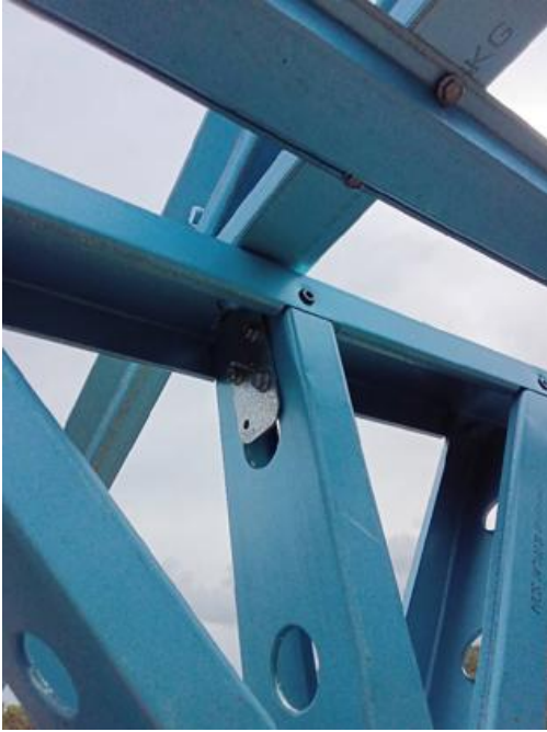
Top plate / truss connection
