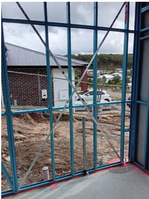
Typical strap bracing
