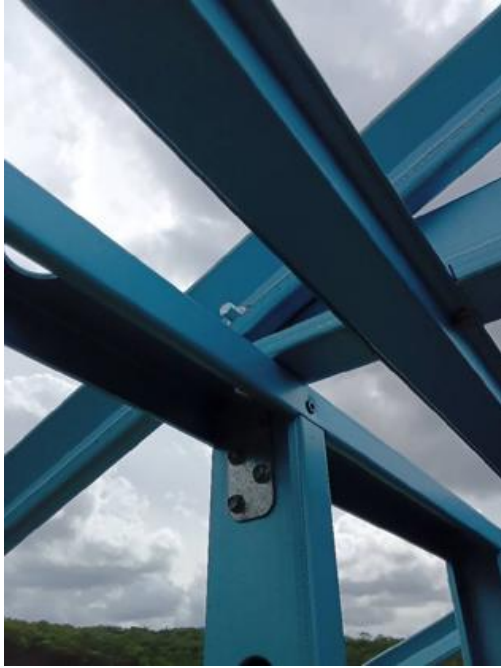
Roof truss tie down
