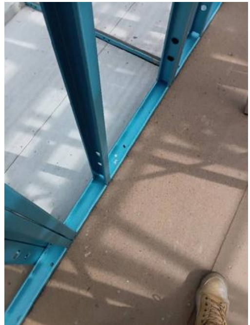
Bathroom wall fixing
