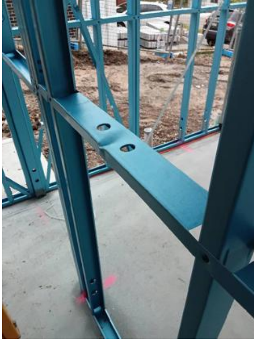
Damaged noggin study
