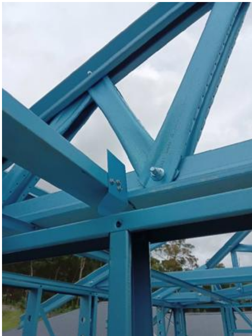
Internal wall bracing
