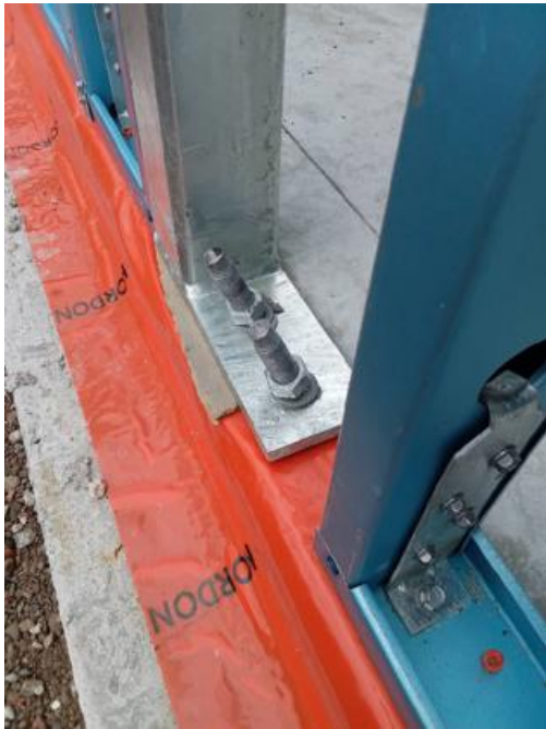
Fixing bolts fixed on an angle
