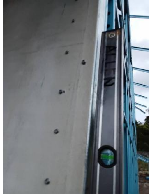
Column out of plumb front right-hand side
