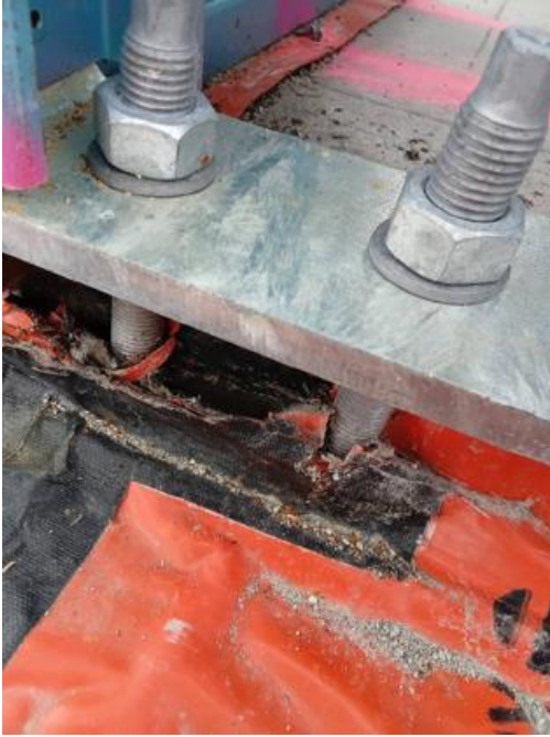
Termite barrier damaged
