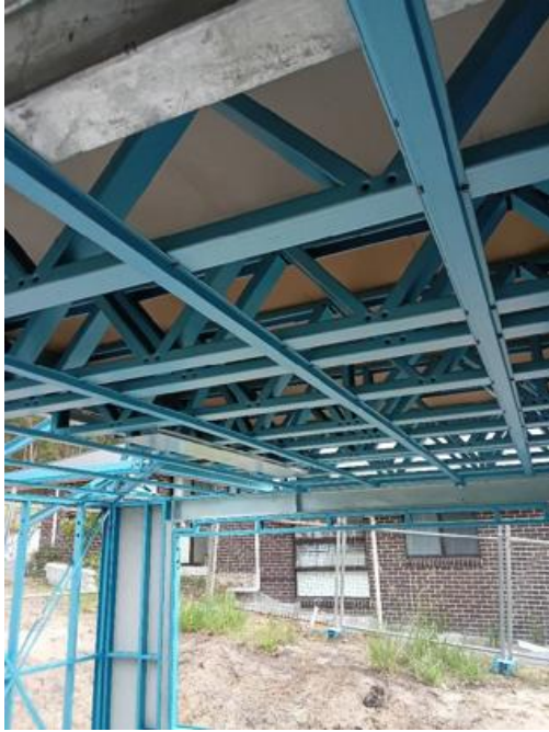
Typical floor framing
